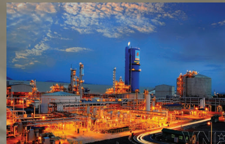
DAM PHU MY FACTORY
